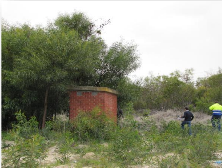
Figure 1 Dense stands of Alien vegetation close to Ankerlig Power Station
